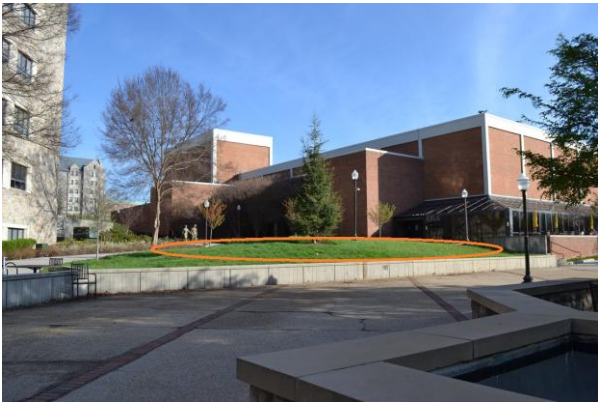
Site view facing Squires from GLC Plaza
